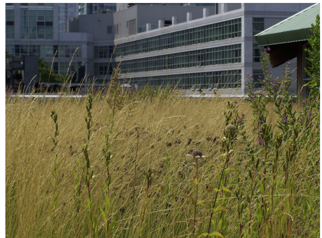
Fig. 2. Green roof on Mountain Equipment Coop, Toronto.
