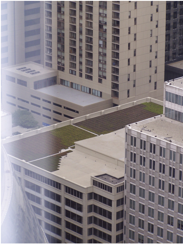
Fig. 3. Sedum green roof on parking garage, Chicago.
