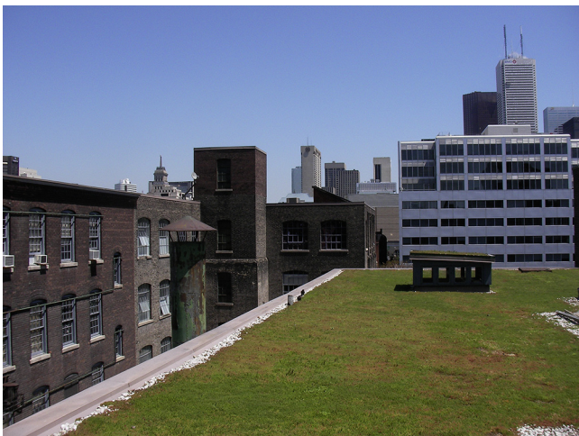
Fig. 4. Green roof on 401 Richmond (flat, sedum or grass-like roof).
