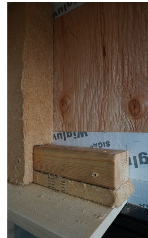
Insulation around window
