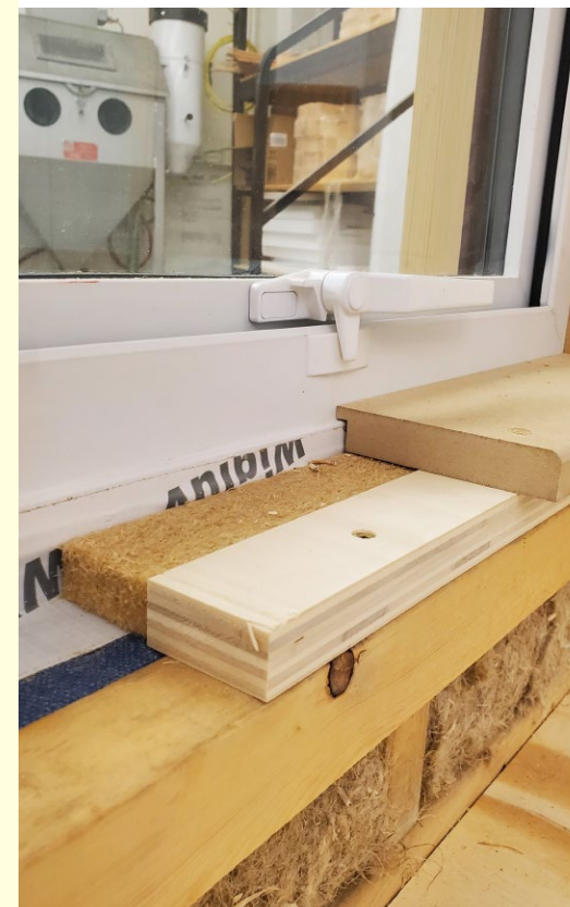
Interior window insulation
