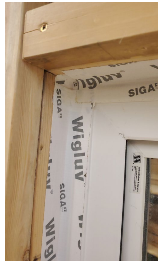
Interior-taped air sealing
