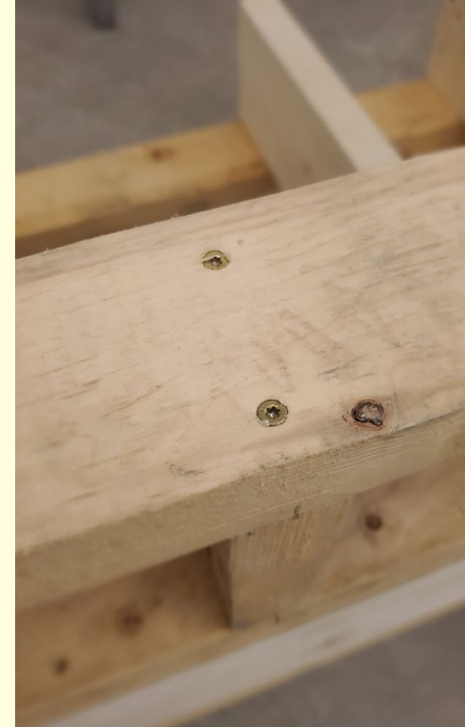
Structure is screwed together
