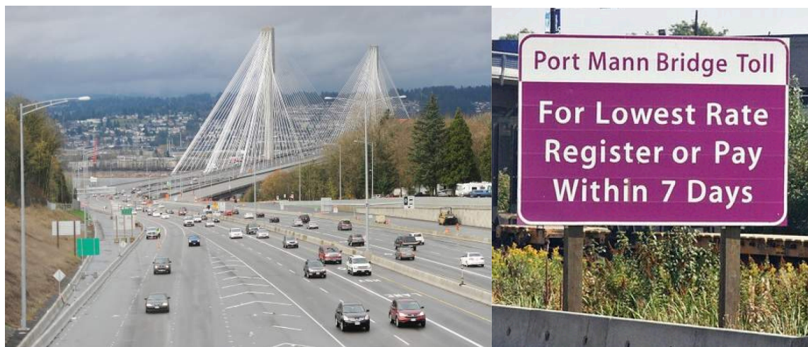
Figure 9: Traffic on the Portmann Bridge, BC Highway 1 (Source: Vancouver Sun)
