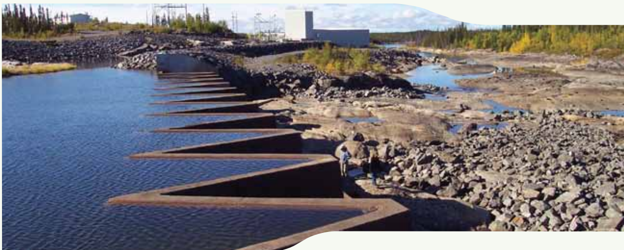
The Snare Cascades spillway.
