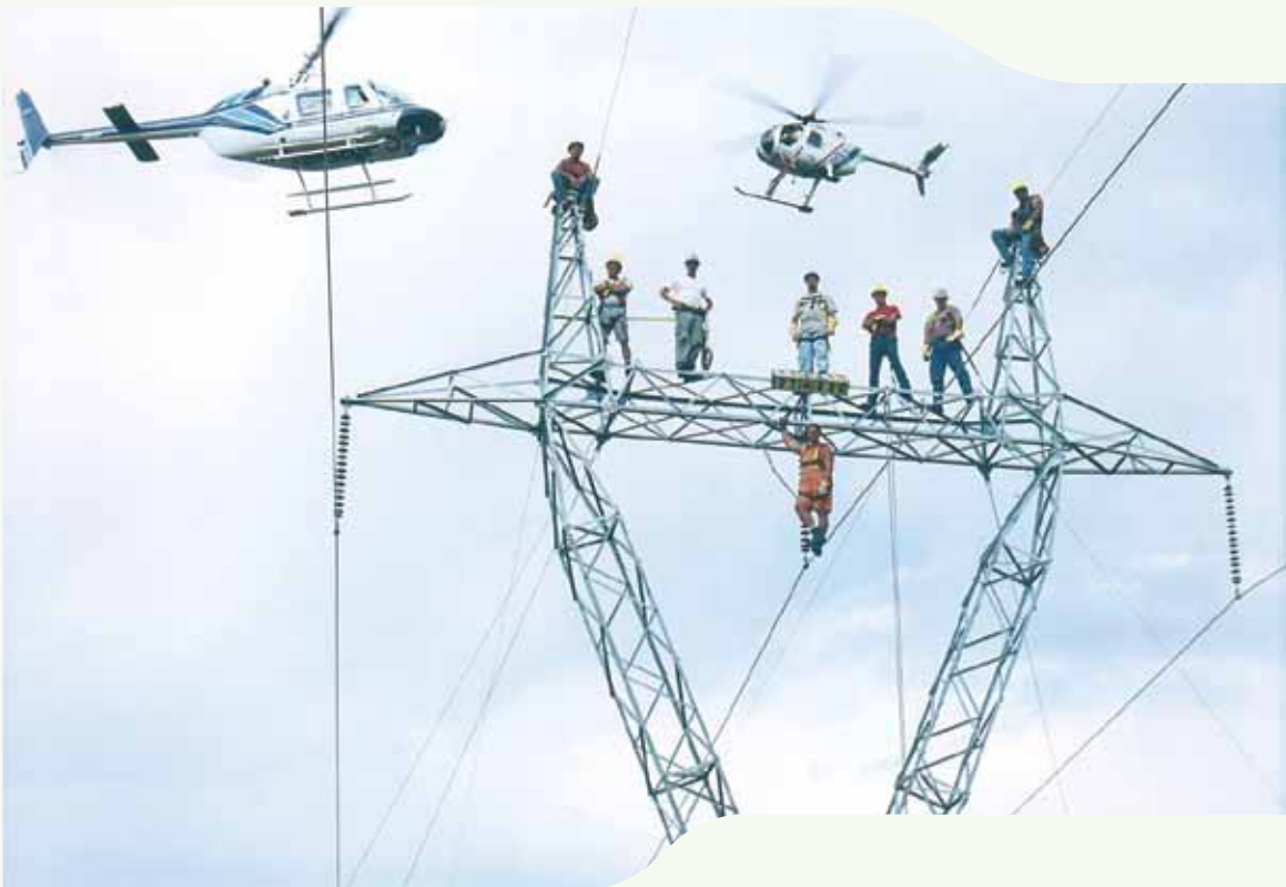
Constructing a transmission line in the NWT.
