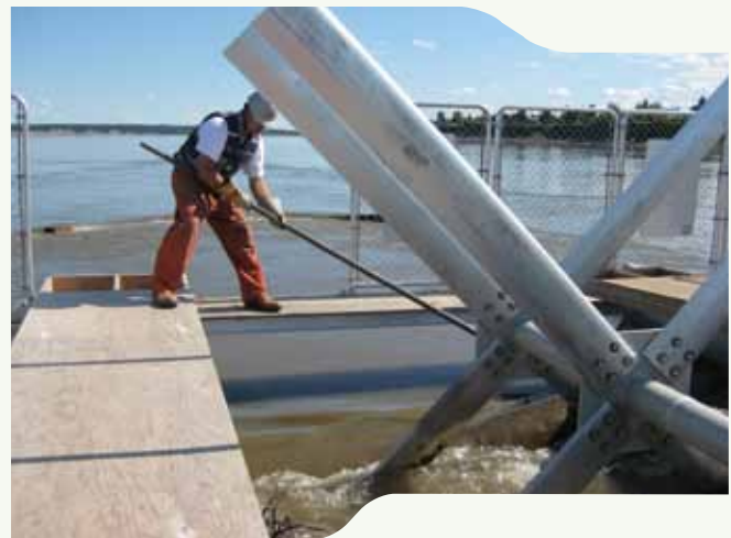
Removing the log that damaged the Fort Simpson hydrokinetic turbine.
