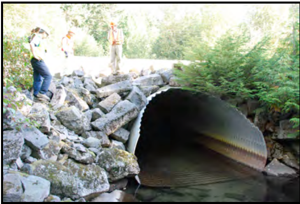
Figure 6: Existing culvert at Millar Creek
