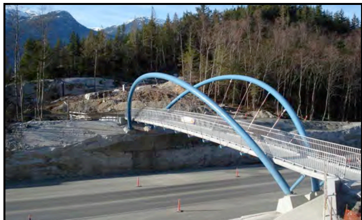
Figure 9: Stawamus Chief pedestrian bridge
