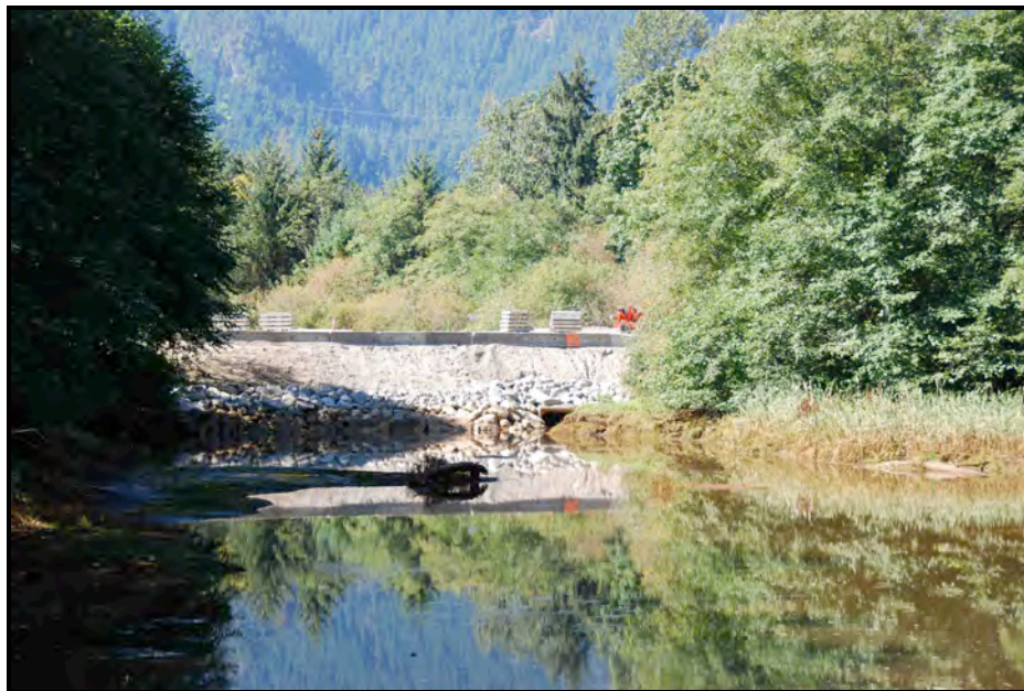
Figure 14: Lowered culvert and tide-influenced pond
