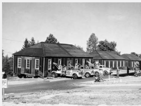
Trucks moving army huts into place on West Mall (UBC Library archives)
