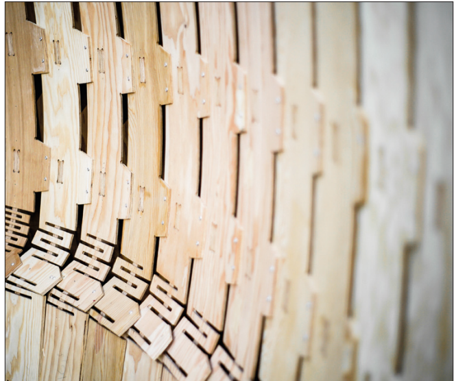
7 Detail of the connections between elements. The stressed skin is formed by vertical plywood strips that connect to each other with flaps, making it possible to bend in a direction other than the strips themselves.
