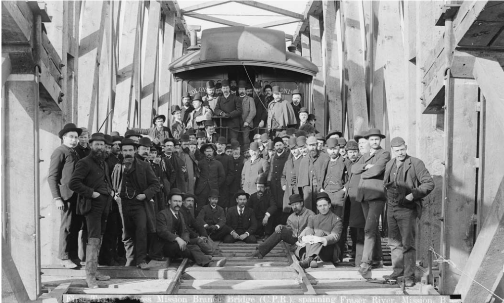
1. First train to cross Mission Branch Bridge (C.P.R.), spanning Fraser River, Mission, B.C., Canada. (Courtesy of City of Vancouver Archives.)
