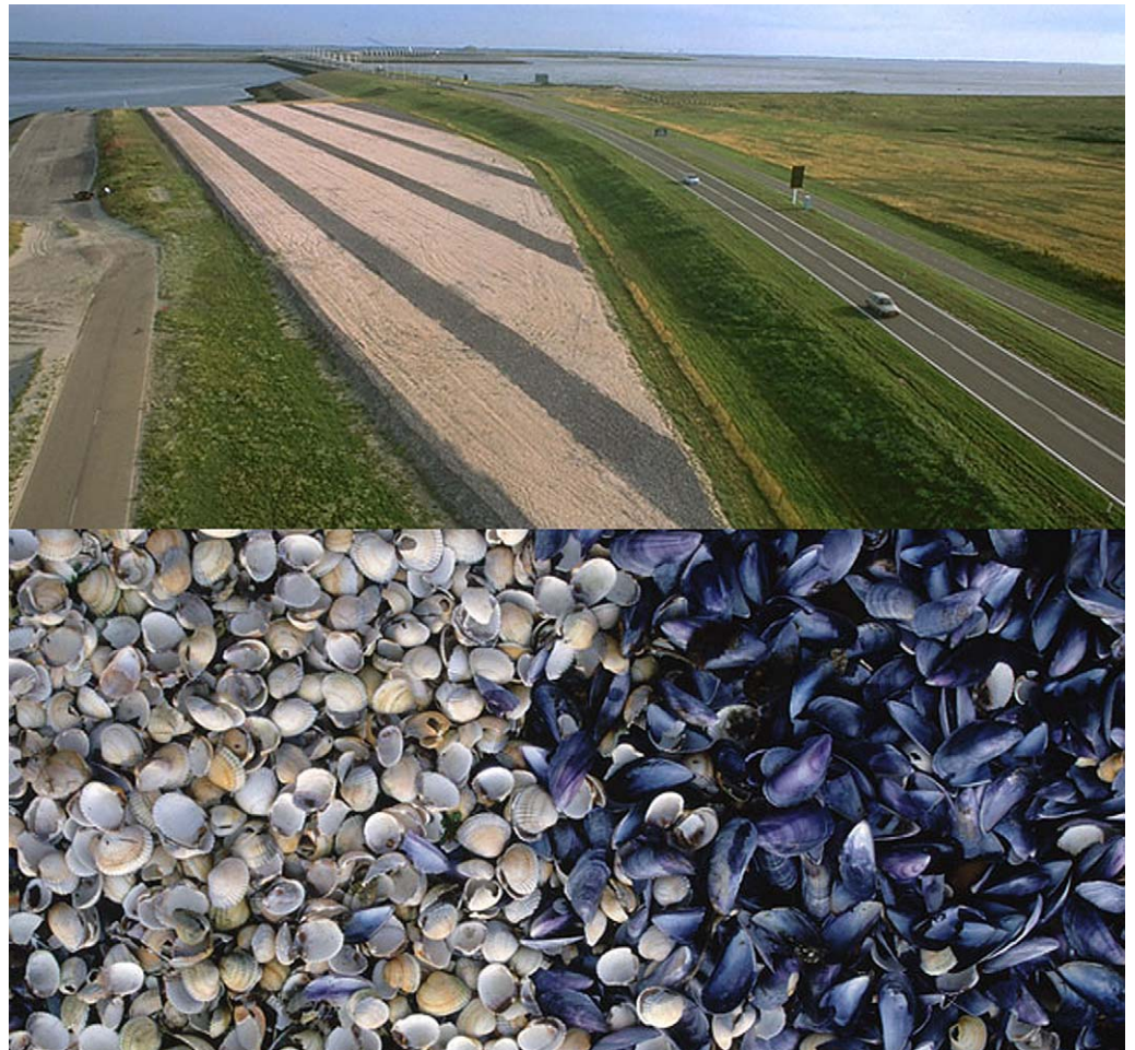
8. West 8’s Eastern Scheldt storm surge barrier design works at a scale suitable to highway speed, but composed of smaller scale shells which also function ecologically as camouflage. (Courtesy of West 8.)
