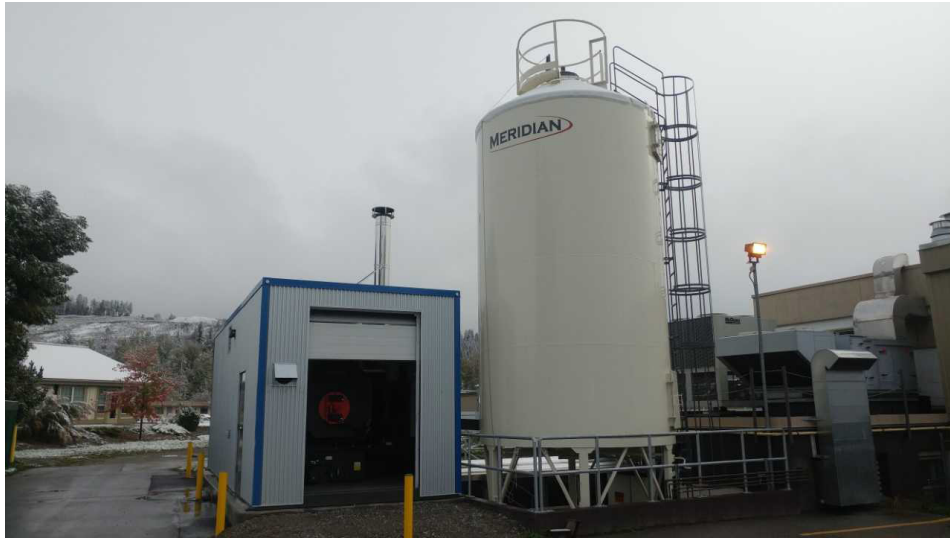
Figure 13. Biomass boiler plant in Golden (2019). Retrieved by Interior Health Authority via 2019 Carbon Neutral Action Report . No changes made. All rights reserved. Generalism and telehealth are also promising strategies in health care practices that can minimize GHG emission. We will discuss this further in Chapter 4 of this compendium.
