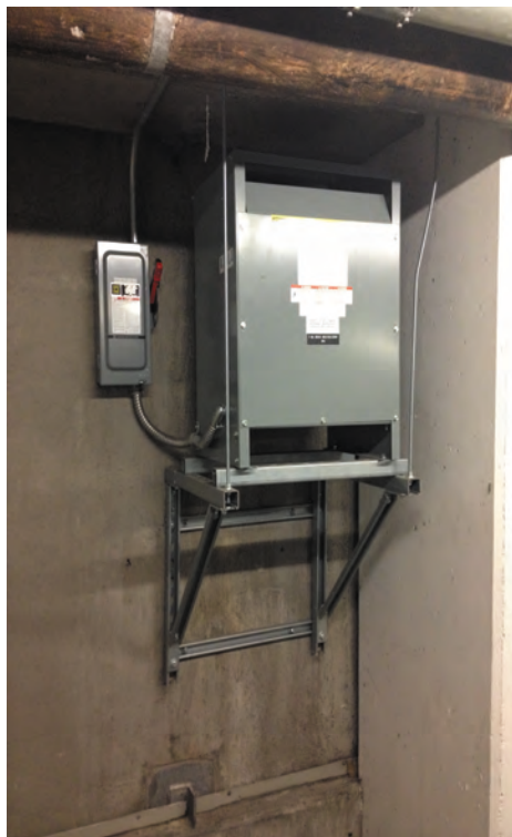
Figure 1: Example of a wall mounted transformer
