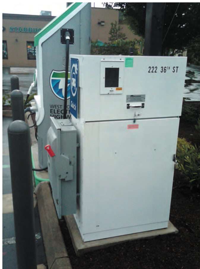
Figure 3: Example of a visual disconnect mounted in a visually obtrusive location, the general public and EV drivers will not need to use this switch, therefore it should be positioned in a less conspicuous location.
