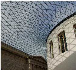
C) Lattice roof truss at British Museum
