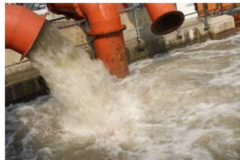
Wastewater outfall. Theepochtimes.com
