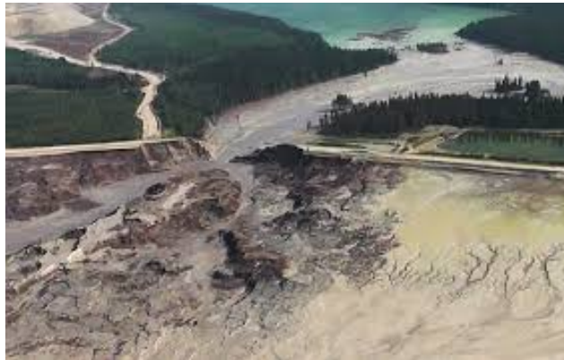
Mount Polley Tailings Pond Breach
