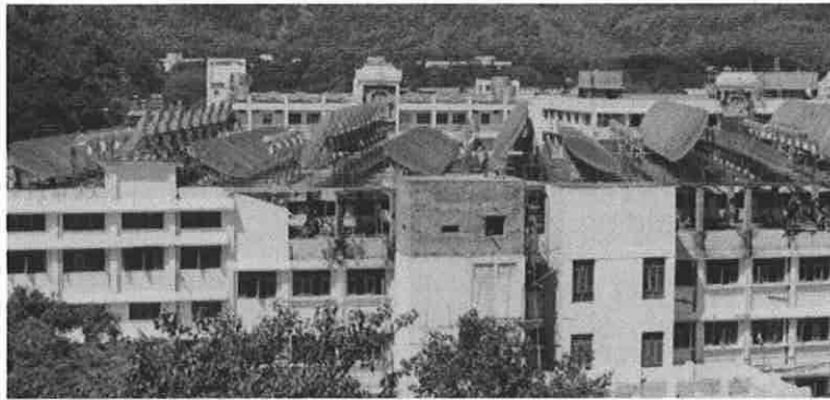
The world's largest, solar-steam cooking system, used to cook for 15,000 people a day, is in Tirumala, India. It has been functioning satisfactorily since October 2002. It generates approximately 4,000 kilograms of steam per day and is expected to save approximately 118,000 litres of diesel fuel per year.
