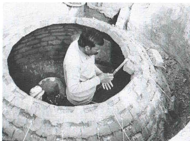
Building a biogas digester
