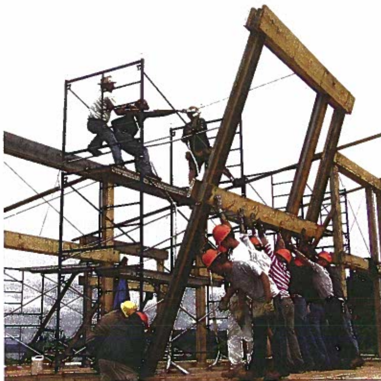
Students of architecture execute experimental wood structures at the Ghost International Architectural Laboratory initiated and directed by Brian MacKay-Lyons in Nova Scotia. The building camp has taken place every summer since 1994. Ghost 7, 2006
