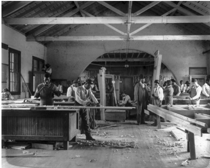
Students constructing a wood roof truss at Tuskegee Institute.
