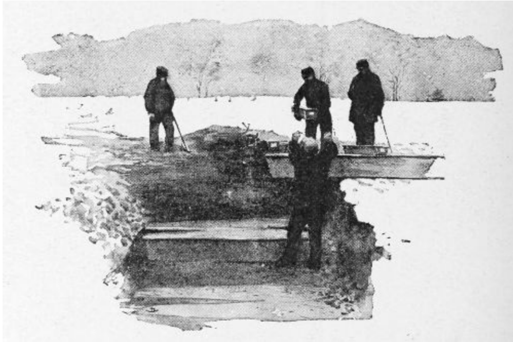
THE TRENCH IN THE POTTER'S FIELD.
