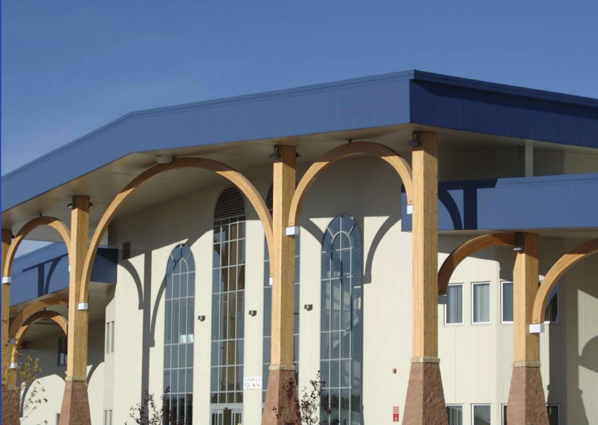
Energetic Learning Campus of North Peace Secondary School
