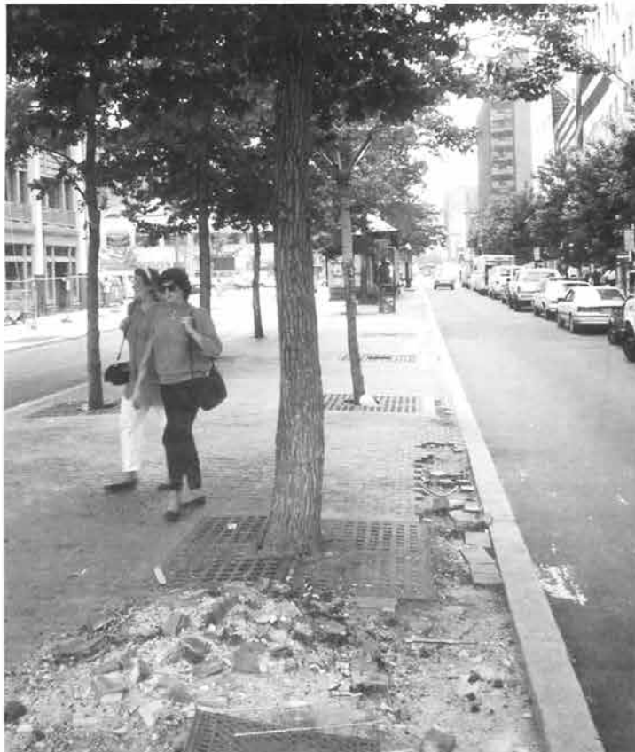
Figure 1.1.2. Lack of understanding of the relationship between tree biology and urban soil often results in either dead trees or dead sidewalks.
