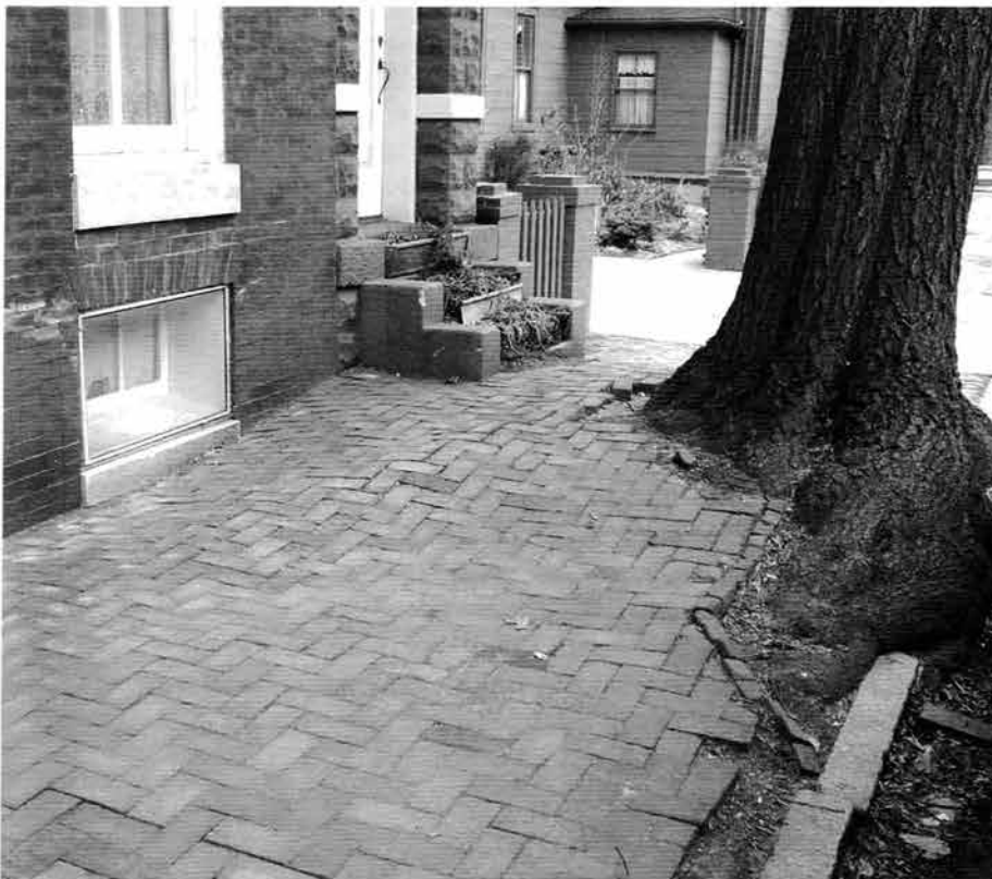
Figure 2.2.7. Mature tree in a small space, successfully altering the paving around its base. Though planted in a 4-foot space, the tree has enlarged the hole many times and lifted the ground almost a foot. Several generations of sensitive landowners have reset bricks to accommodate the tree's needs. Unfortunately, not everyone is this considerate.
