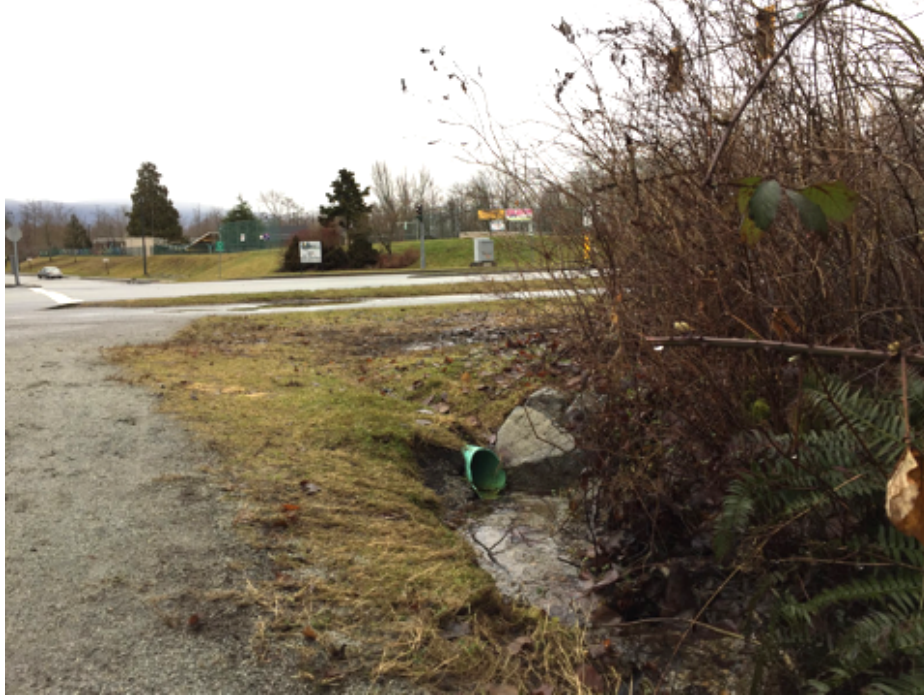
Picture 1: a stream-road crossing tube near the headwater of the stream
