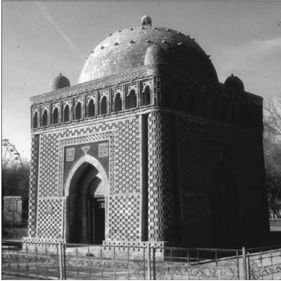
Fig. 5. Mausoleum of Isma'il the Samanid, Bukhara, Uzbekistan, 914-943 AD. (Author, 1997)
