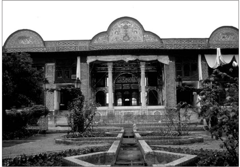
Fig. 4. Narenjestan Qajar summer residence, Shiraz, 1881, renovated 1960s. (Author, 1999)
