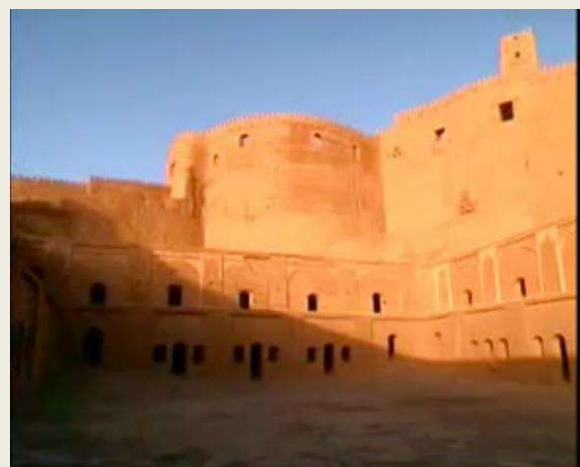
Fig. The Barracks, Stables and the Quarter of the commanding generals
