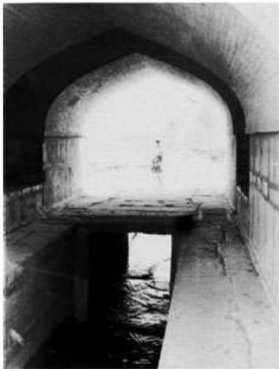
Pl. VIa. Water channel under the bridge with the sluice-gate.
