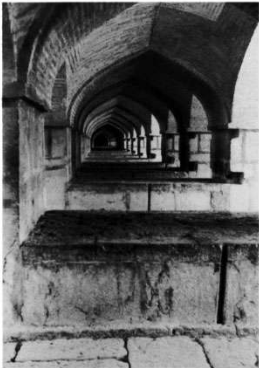
Pl. VIb. Longitudinal view under the bridge from south to north.
