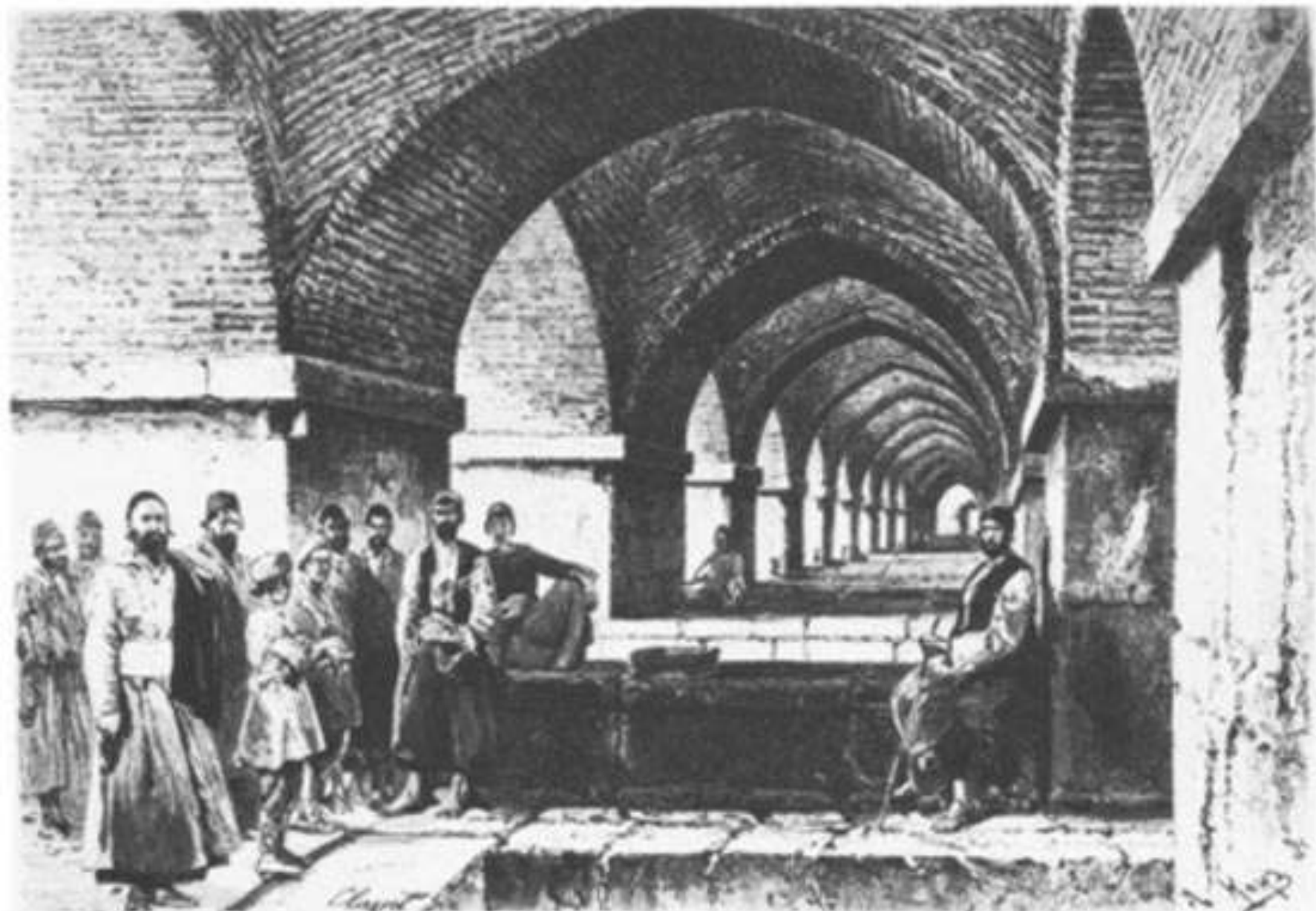
Pl. IIIb. Vaults of the Pul-i Khwājū. Drawing in Jane Dieulafoy, La Perse , 1887.
