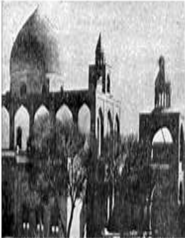
Exterior view of Vank Church and its free-standing belfry
