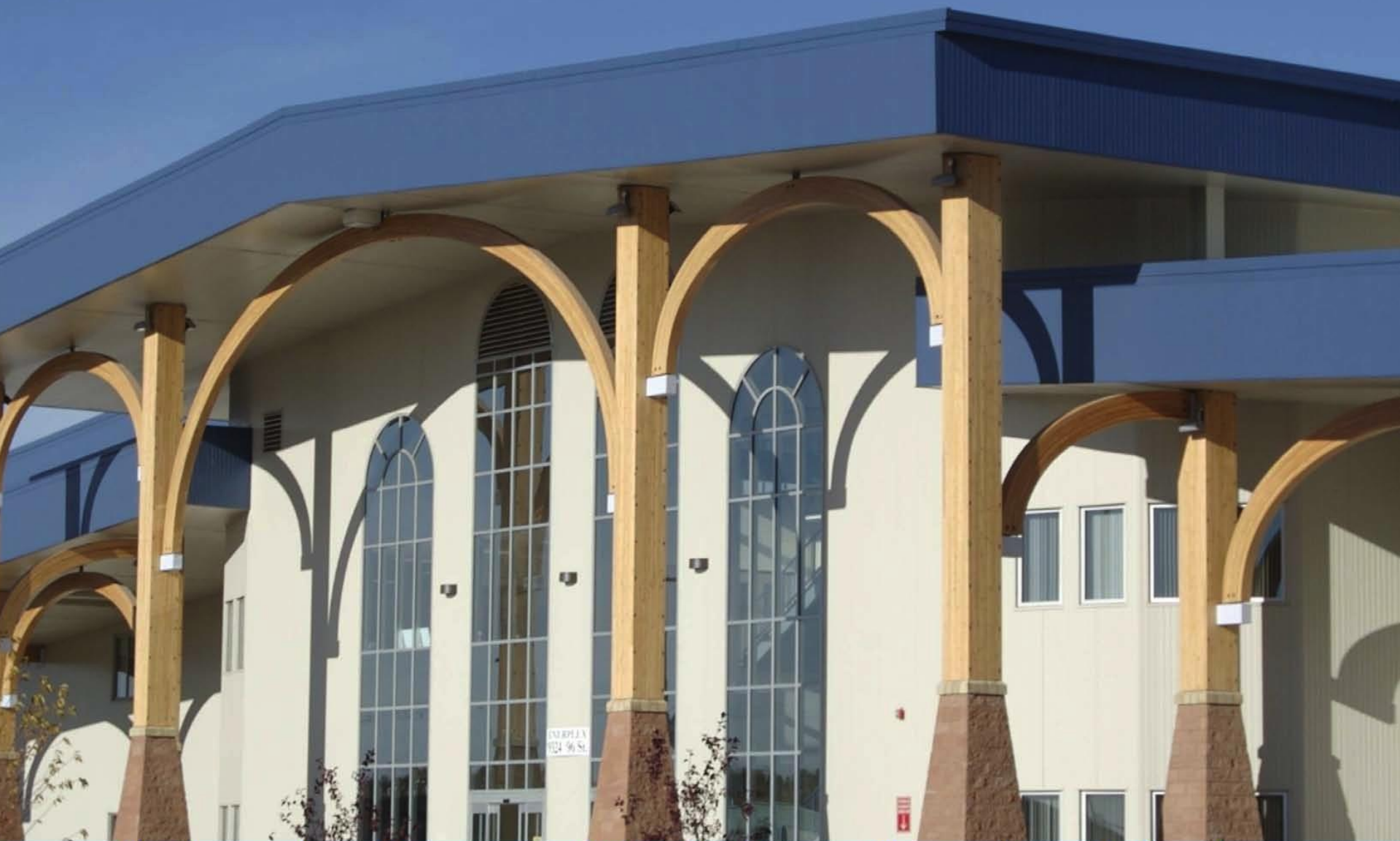
Energetic Learning Campus of North Peace Secondary School
